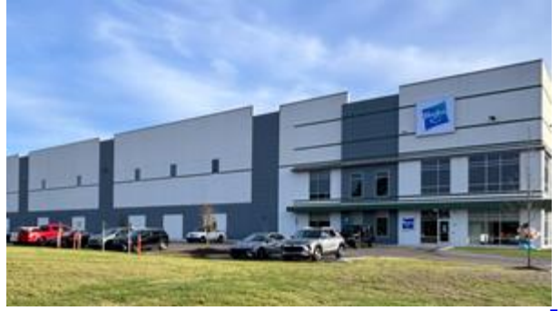
The 600,000-square-foot distribution center is located in Midway, Georgia
